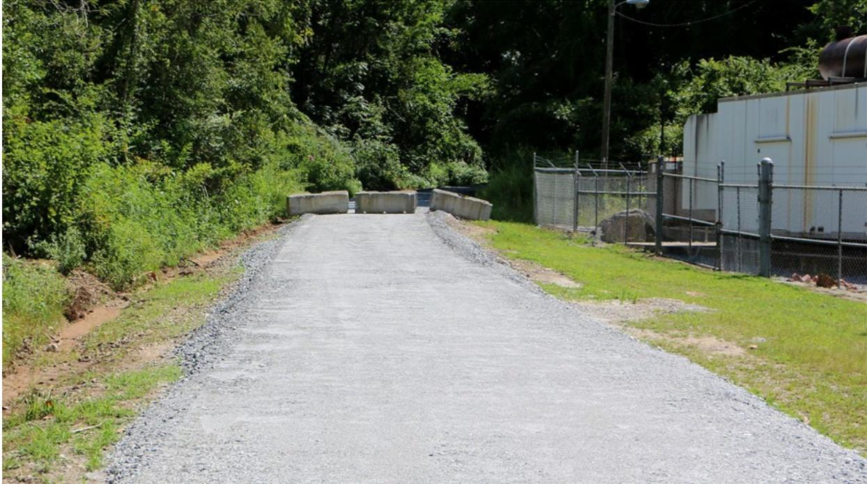
*The City of Lenoir Public Works Department has placed stone base on the Rail Trail in preparation for paving. The City plans to pave the Rail Trail from North Main Street to Willow Street and possibly all the way to Harper Avenue.*
